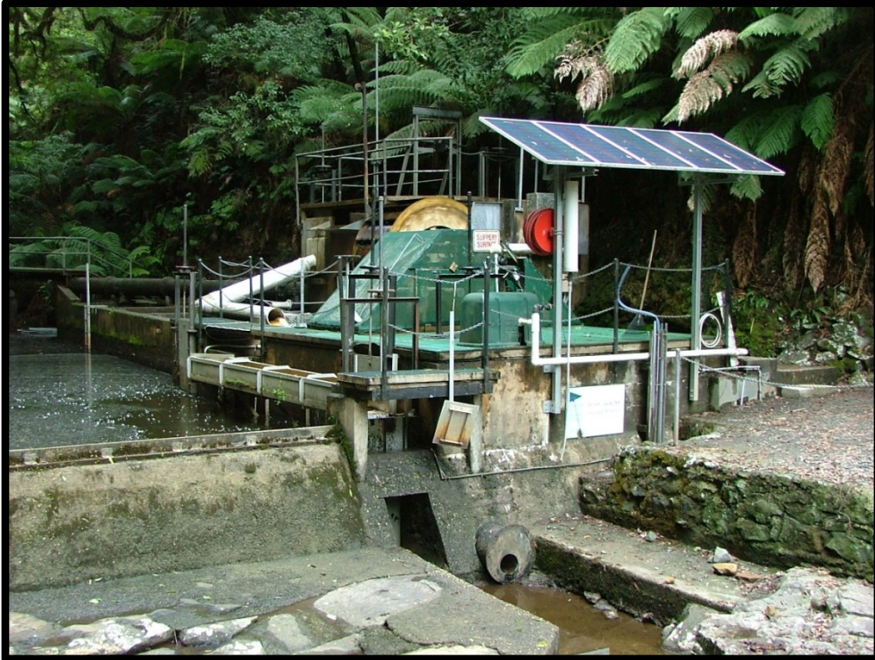
One of the Arkins Creek diversions high in the catchment that gravity feeds water to Warrnambool.
